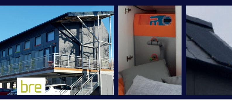
These innovative living spaces offer a low cost, prefabricated super energy-efficient micro home that maximises land held by a landowner making it multi-functional. The modular home building Zed Pods in this project designed unique, small footprint, highly insulated homes that sit on stilts above car parks that allow cars to park underneath.
